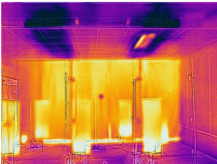
Thermal image showing heating and cooling sources in the test rig.
